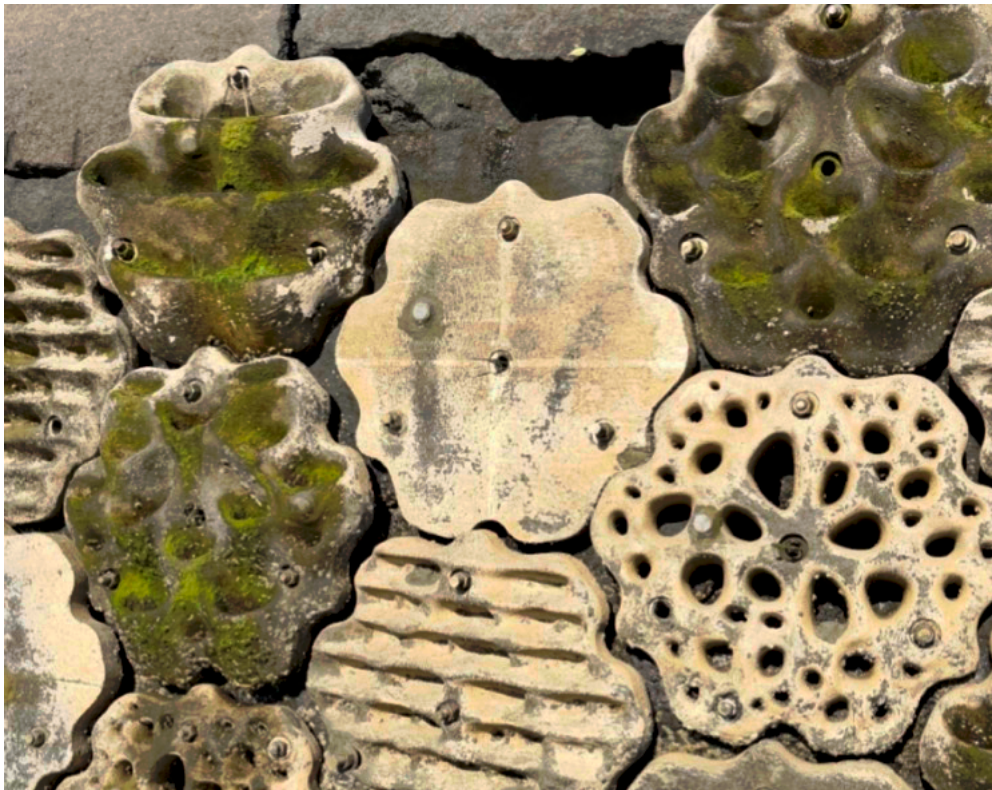
Figure 19: Condor Street Urban Wild in June 2026. Note the extensive green algae around rockpools, although the control and other panels have not recovered as well.
