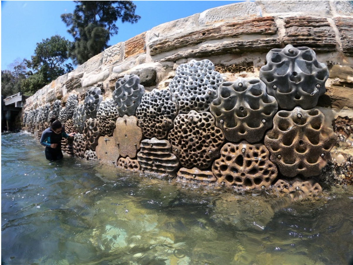
Figure 1: An early Living Seawalls installation in Sydney Harbor, Australia. (Image credit: Alex Goad).
